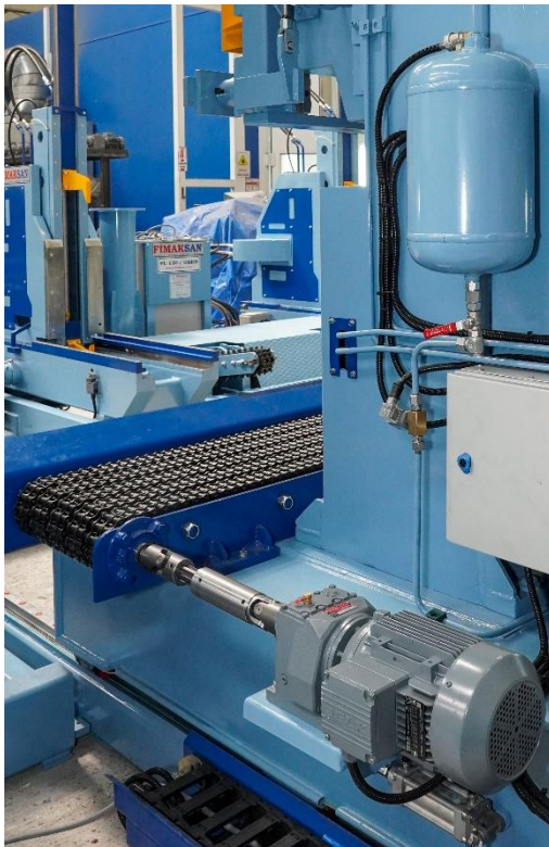
Sawn board & sawdust Removal chain
